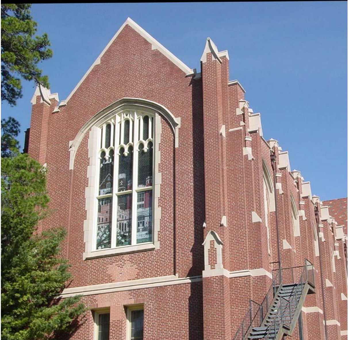
Photo 15.16 Proper Gable/Pier Design
